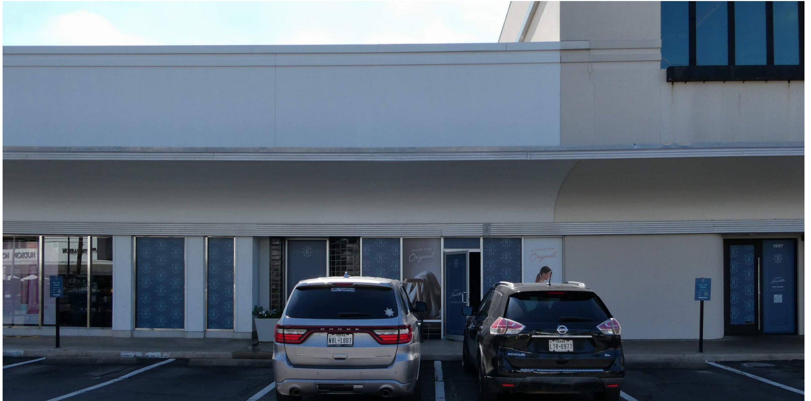
Existing Building Photo
